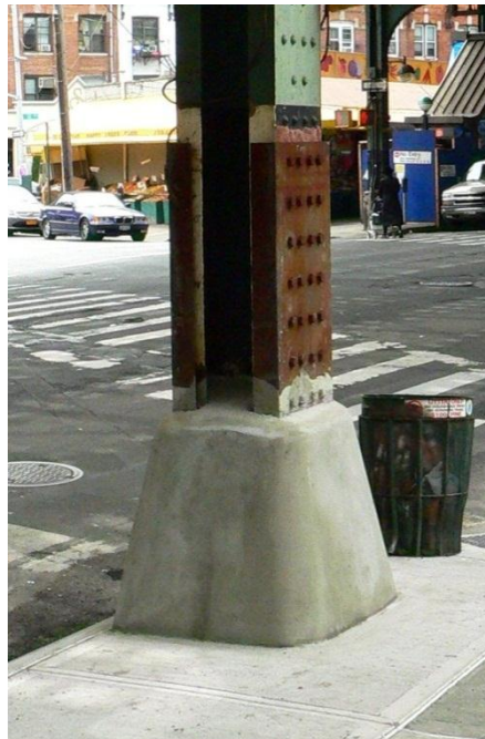
Figure 7: Concrete-Covered Column Base
