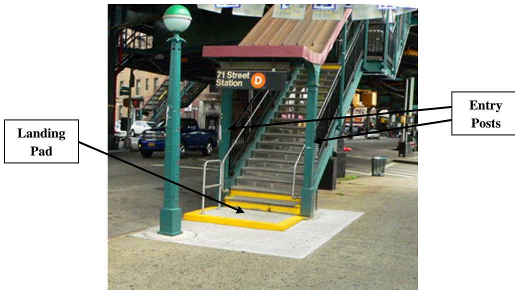
Figure 6: Example of entry posts and landing pad at a station entrance.
