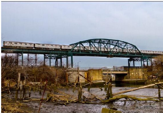
Bronx River Truss Bridge
