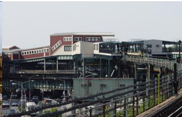
High Elevated Structure: Broadway Junction Station
